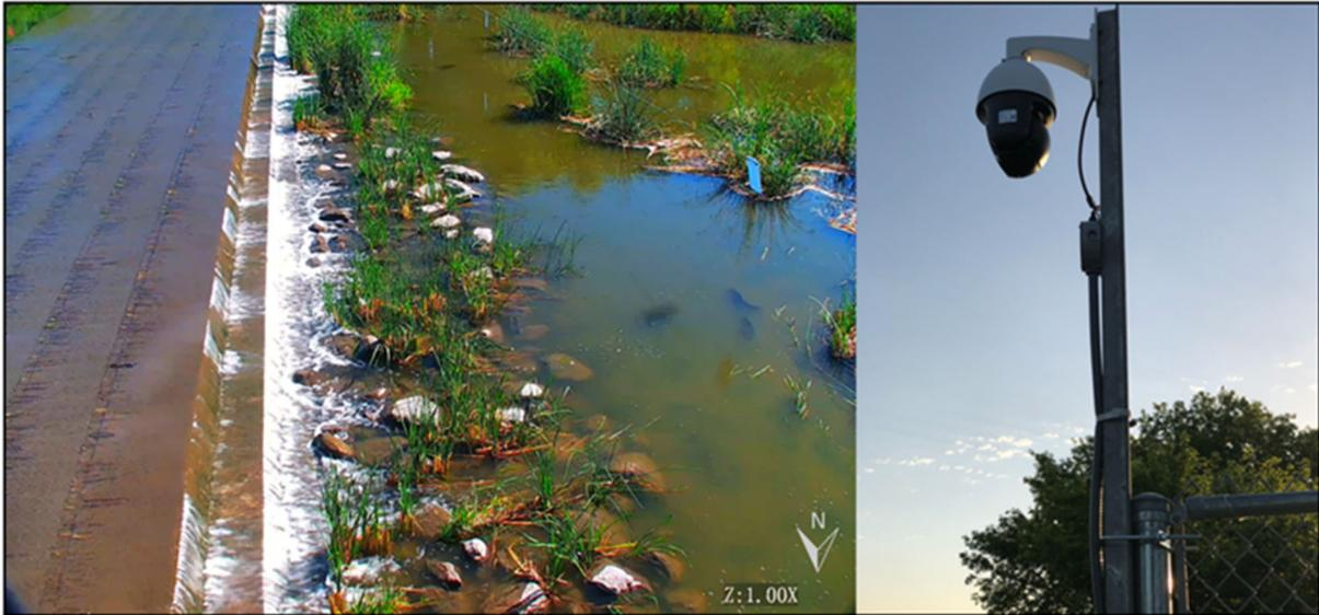
Figure 15. Outdoor video surveillance camera (Sunba network PTZ) installed above the electric fish barrier at the outlet of Lower Gar Lake on June 14th, 2022. The camera is positioned to allow for the best possible view of fish movements on the north side of the barrier.
