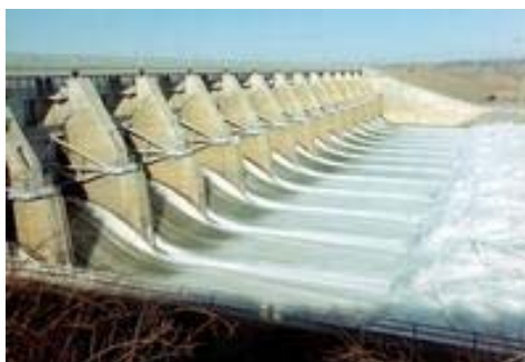
Gavins Point Dam
