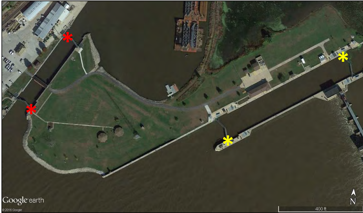
Figure 1. Locations where stationary ARIS imagery will be collected in the main chamber (yellow) and auxiliary chamber (red) of Lock 14.
