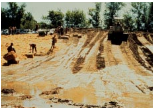
Figure 7. The raising of this federal agricultural levee during the 1993 “flood fight” threatened neighboring lands by further constricting the floodplain and forcing flood waters to higher elevations. Photos courtesy of the U.S. Fish and Wildlife Service.
