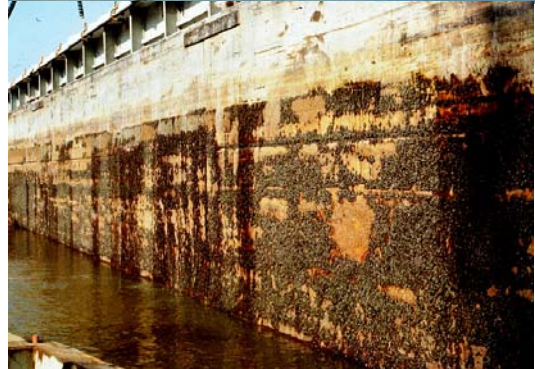
Figure 4. View of an Upper Mississippi River barge fleet and closeup of a barge hull literally covered with zebra mussels.
